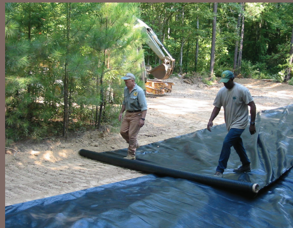
Geo-textiles used to strengthen road base and prevent loss of road material
