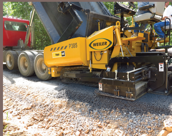
Placing gravel aggregate with a paver
